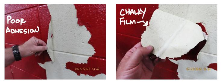
We must make sure that our painting contractor performs an adhesion test on the existing paint <u>and</u> the new paint to the existing paint.
